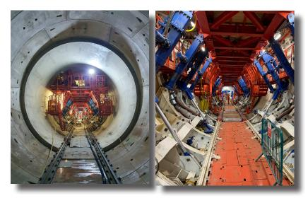
London's new super sewer hits another milestone following the completion of the final section of secondary lining.
