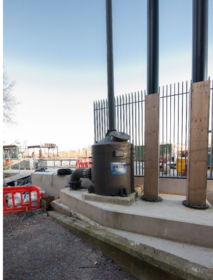
Fence installation behind carbon filter and vent columns
