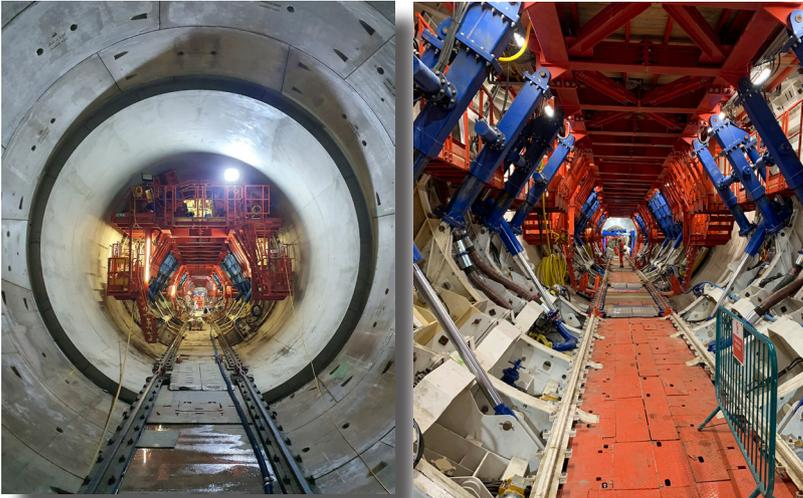
London's new super sewer hits another milestone following the completion of the final section of secondary lining.
