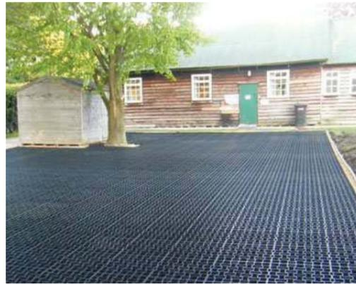
Figure 8.43: Access road ground reinforcement
