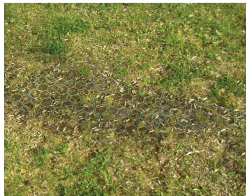
Figure 8.49: Access road grass reinforcement
