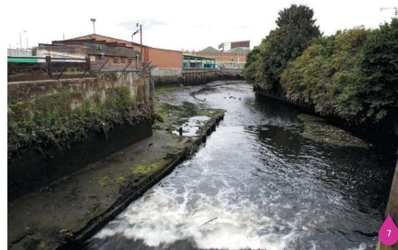
Figure 10.11: Floodwall of Bell Lane Creek
