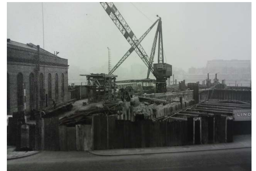
Figure 17.24: Historic photo of Heathwall Pumping Station under construction
