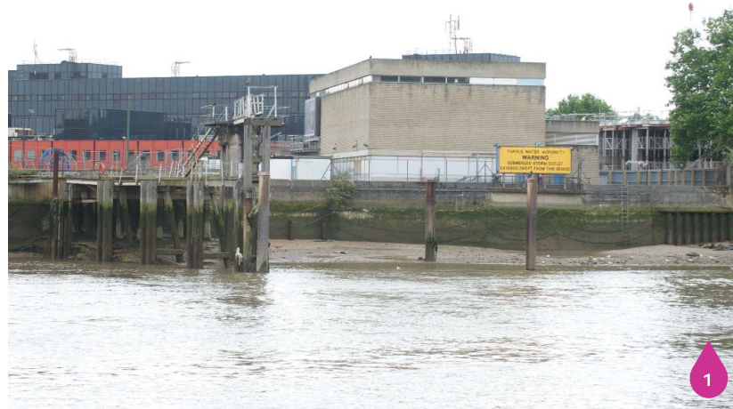
Figure 17.3: Heathwall Pumping Station from the Thames
