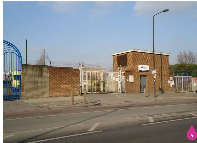
Figure 17.6: Middle Wharf entrance gates and sub-station from Nine Elms Lane
