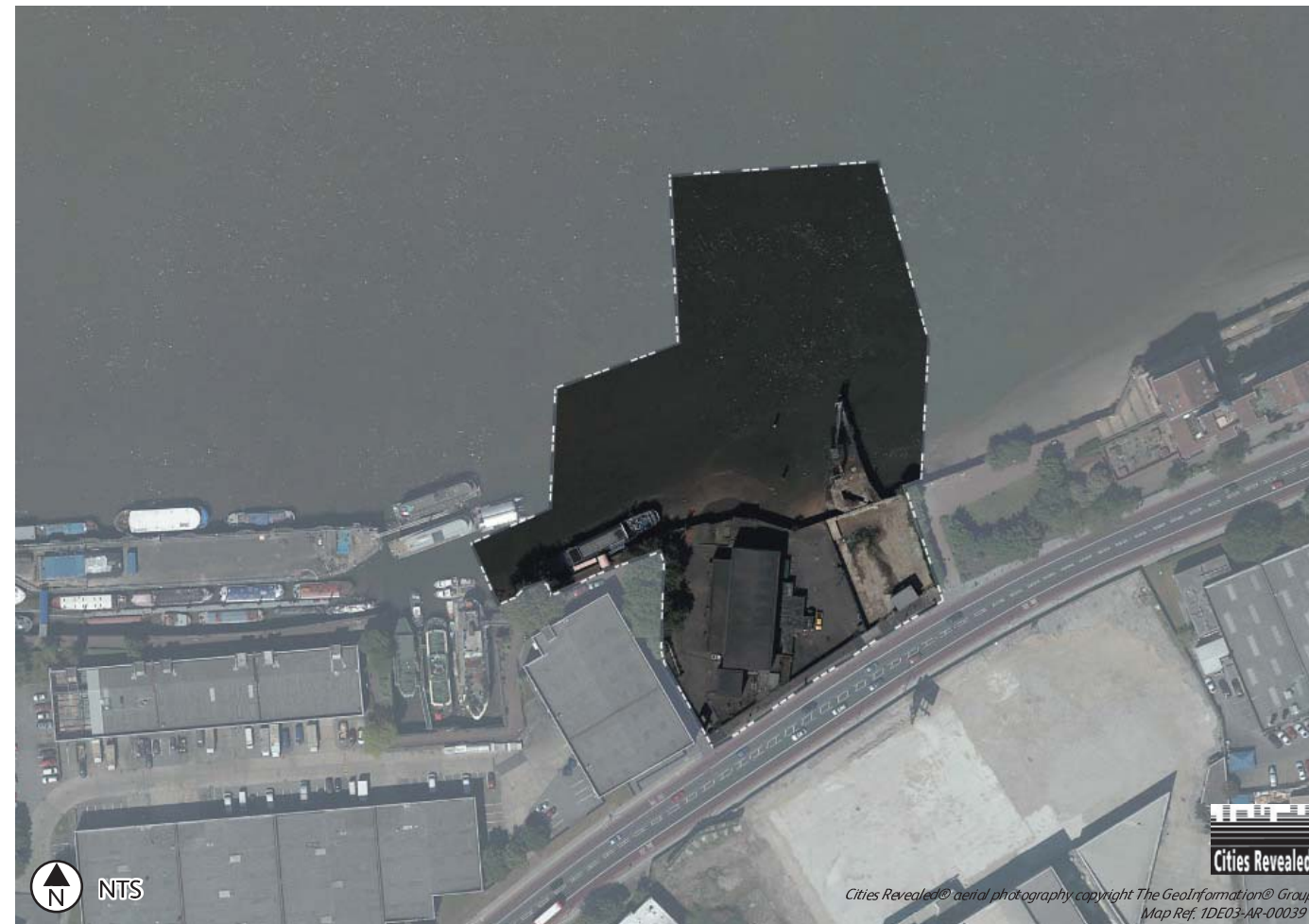
Figure 17.1: Aerial photograph of the existing Heathwall Pumping Station site with LLAU indicated
