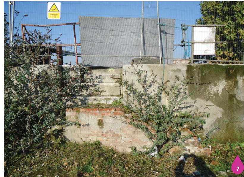
Figure 17.10: Steps to jetty from Middle Wharf
