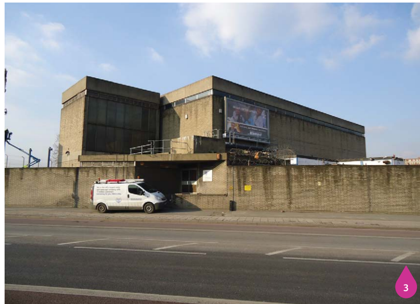
Figure 17.5: Heathwall Pumping Station from Nine Elms Lane
