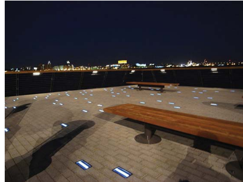
Figure 17.46: Example of in-ground luminaires
