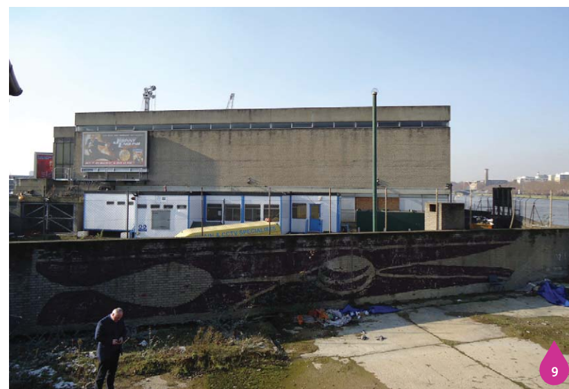
Figure 17.12: Heathwall Pumping Station from Middle Wharf
