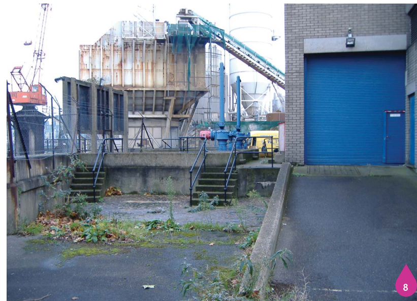
Figure 17.11: Valve chamber and loading bay to the north of Heathwall Pumping Station
