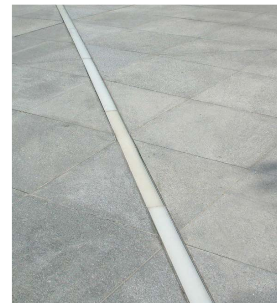
Figure 17.49: Example of in-ground luminaire fitting
