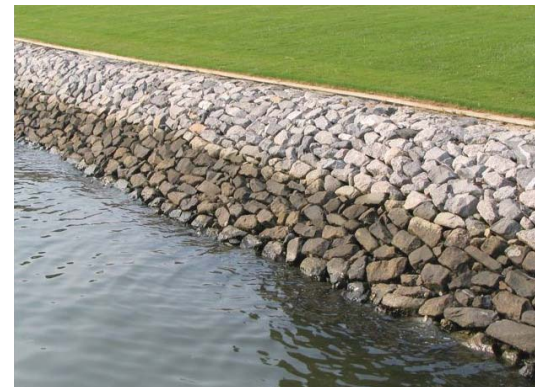
Figure 17.42: Example of 'rip rap' scour protection
