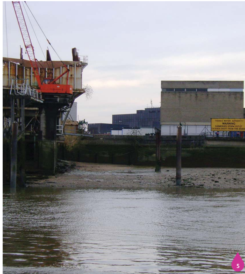
Figure 17.8: River wall and jetty at Heathwall Pumping Station from the Thames
