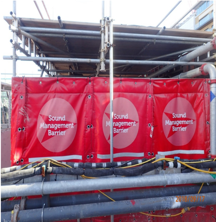
Acoustic enclosure around compressors
