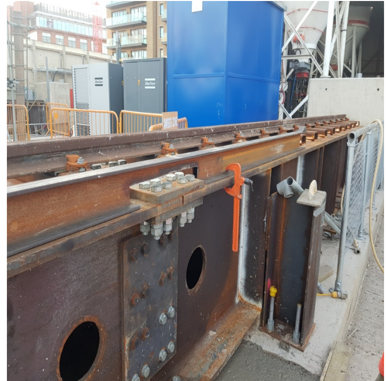
Gantry crane with fully welded rails
