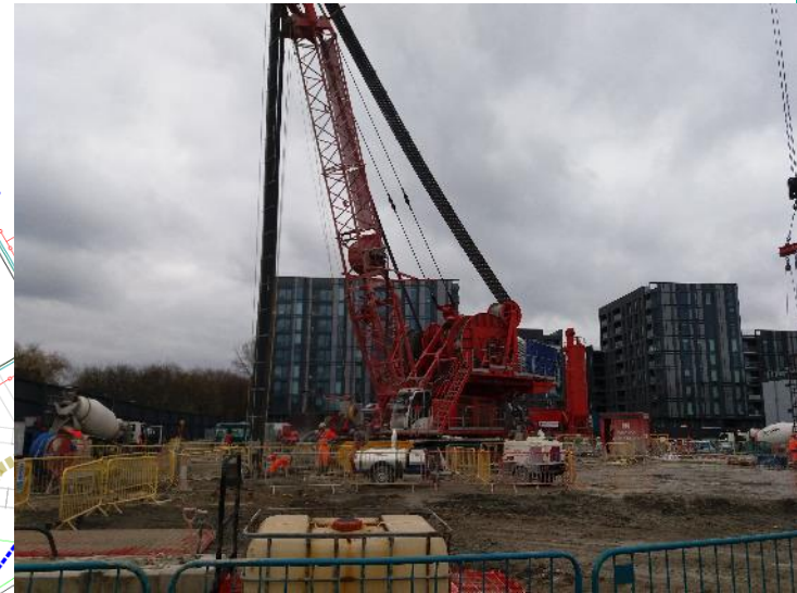
Diaphragm wall construction
