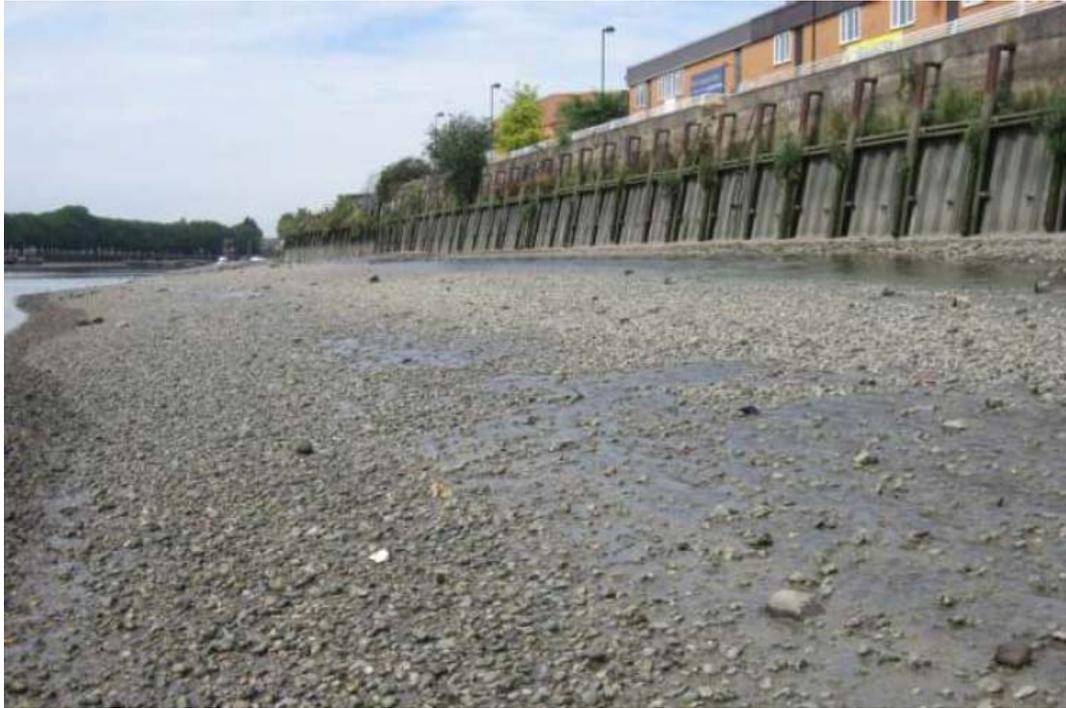
**Figure 8-2 View of foreshore at the location of the works, looking upstream, showing granular surficial sediments. (Photograph provided by HRW)**
