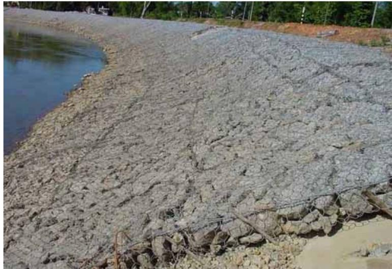
**Figure 5-3 Gabion basket slope protection**
