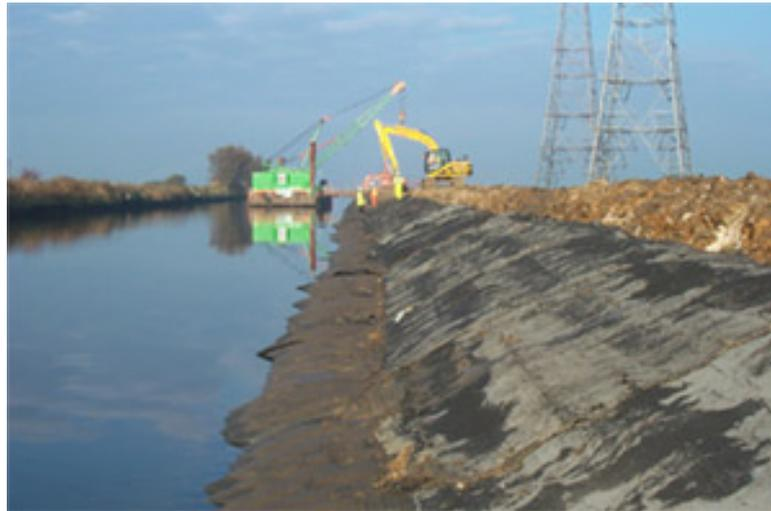
**Figure 5-6 Open stone asphalt erosion protection**
