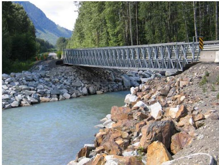
**Figure 5-2 Rip rap scour protection around bridge abutments**
