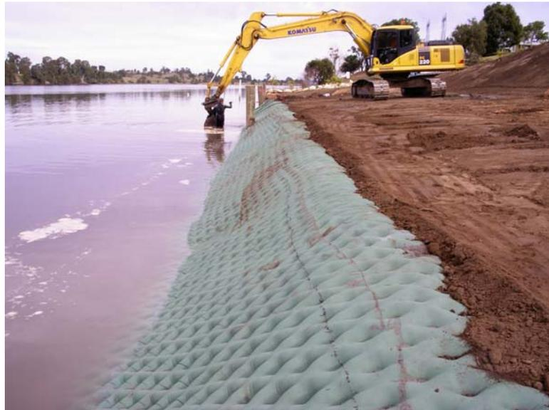
**Figure 5-5 Concrete mattresses for slope protection**
