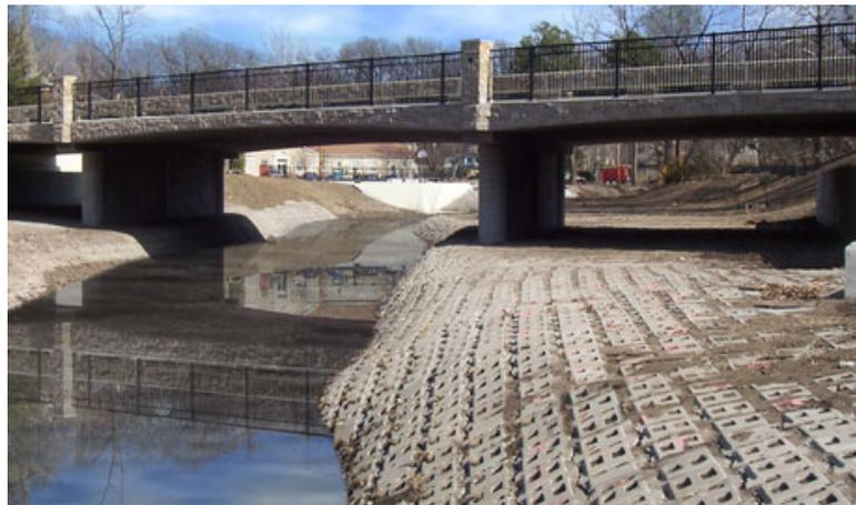
**Figure 5-4 Articulated concrete blocks for slopes and bridge abutments**
