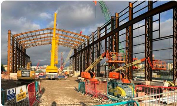
**An acoustic shed is being built at Tideway's site in Fulham to keep noise and dust to a minimum.**
