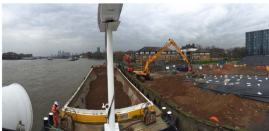
Removal of waste material from Chambers Wharf.
