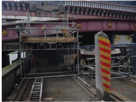
Removal of stairs at Blackfriars.
