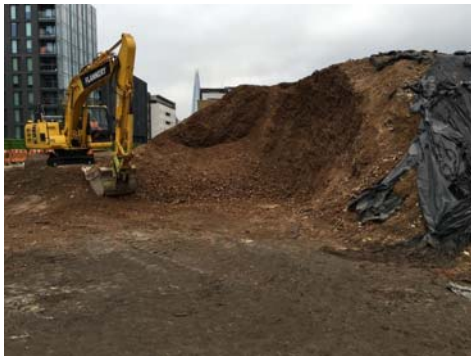
Removal of waste material from Chambers Wharf.
