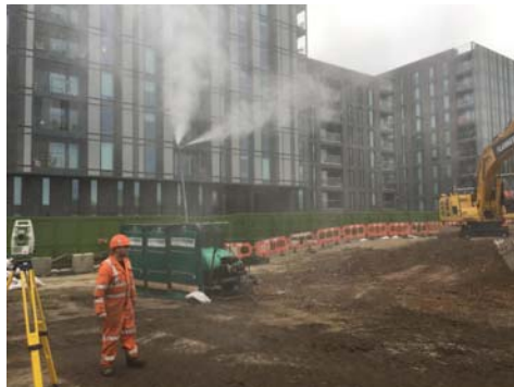
Dust Suppression mist spray at Chambers Wharf
