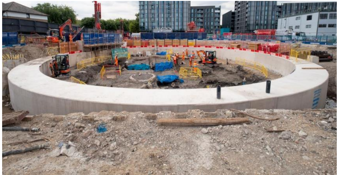
Example of a capping beam at the top of a shaft
