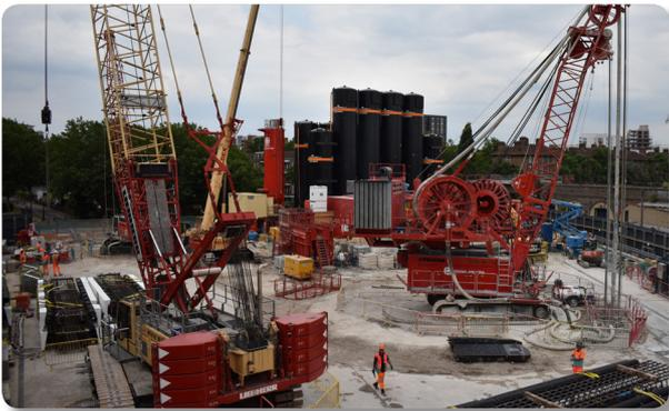
A giant machine called a 'hydrofraise' (pictured) was used to excavate the ground and create each of the 26 shaft wall panels to a depth of more than 60 metres.
