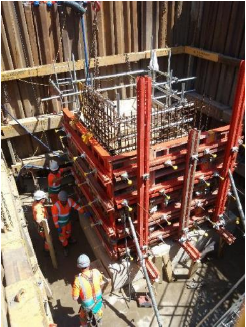
Gallery walls under construction
