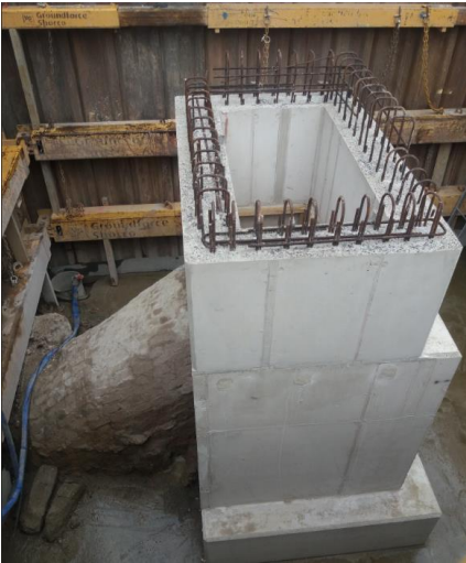
Structure Complete prior to backfilling
