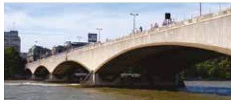
Waterloo Bridge, designed by Sir Giles Gilbert Scott and opened in 1942. Also called the 'Ladies Bridge' as it was partly built by a female workforce, during WWII.
