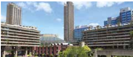
The Barbican Centre, Golden Lane, an arts centre and social housing development designed by Chamberlin, Powell and Bon and completed in 1982.
