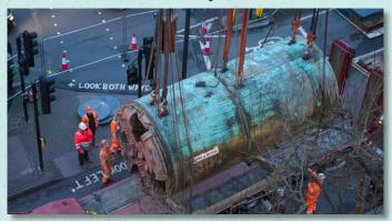
As part of the operation the southbound lane of Putney Bridge was closed for 24 hours to allow a large crane to remove the weighty piece of kit. The team managed to 'lift and shift' the pipejacking machine from the foreshore onto a lorry, where it was then driven to begin its life on another construction project.
