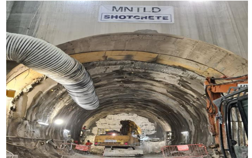
An example of a tunnel adit being constructed
