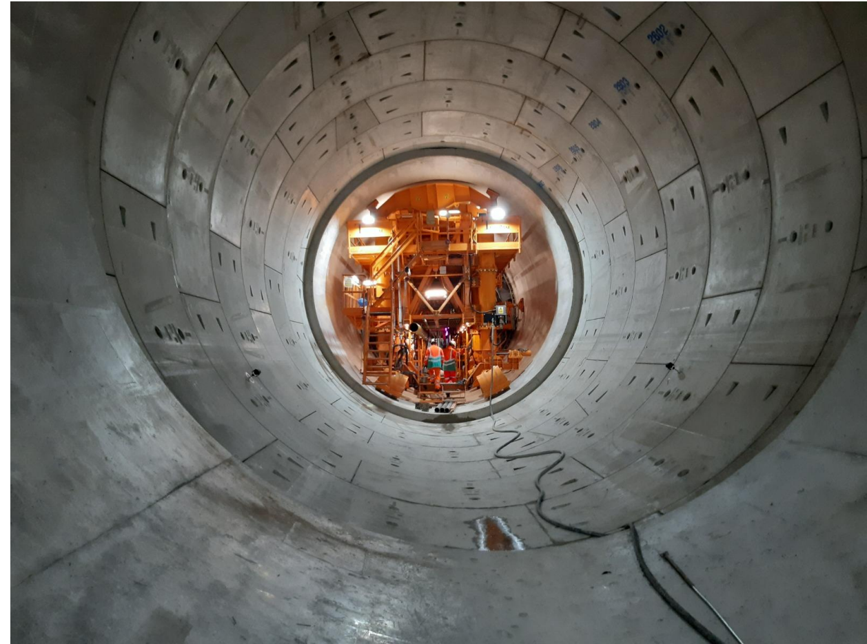
Secondary Lining - Concrete Shutter
