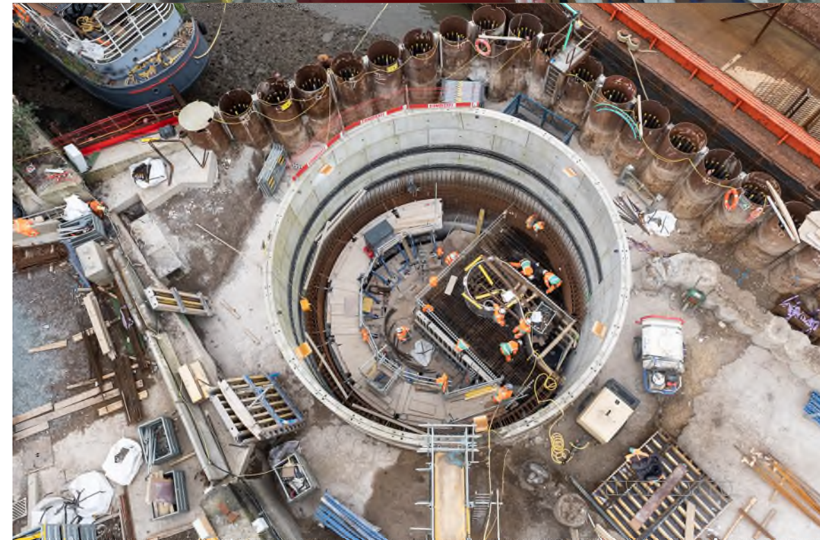
HPS Shaft Secondary lining & Internals
