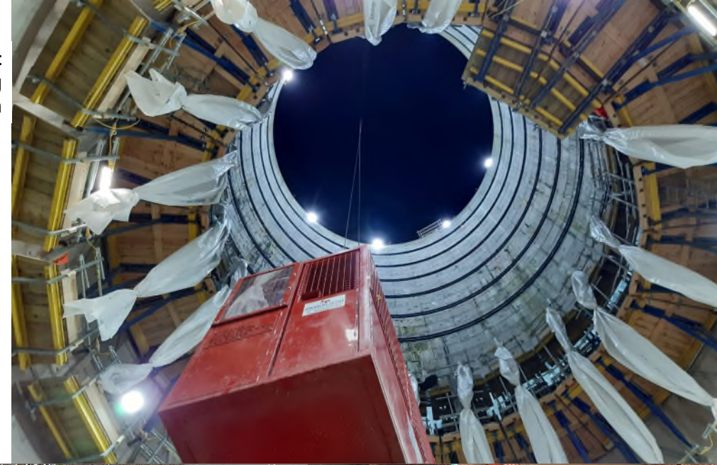
CSO shaft secondary lining jumpform
