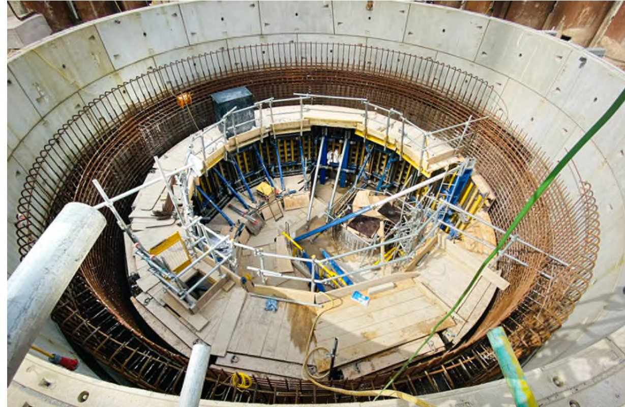
Shafts' secondary lining steel reinforcement delivered via River
