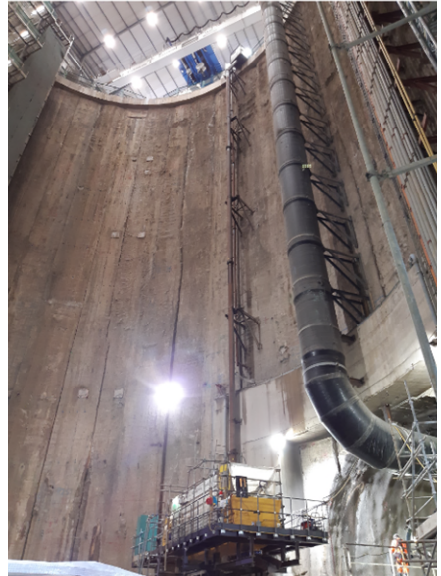
Gravity used to transport secondary lining concrete down shaft
