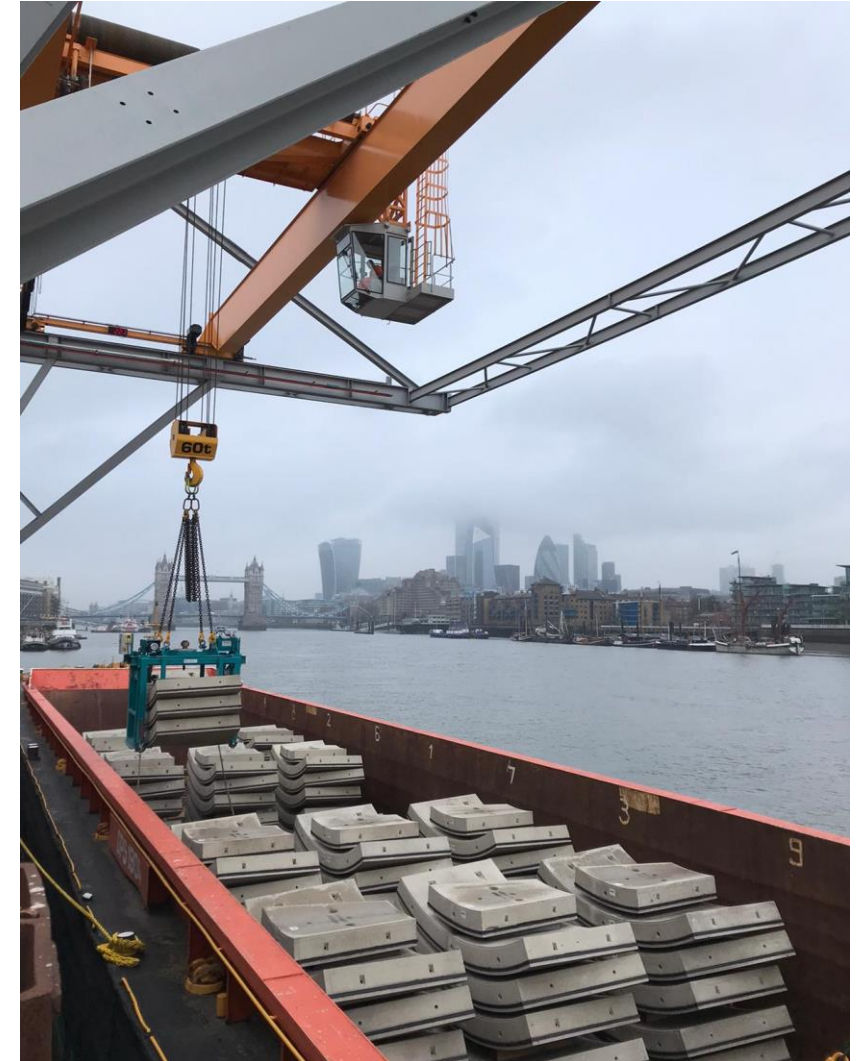
Tunnel Ring Delivery by River
