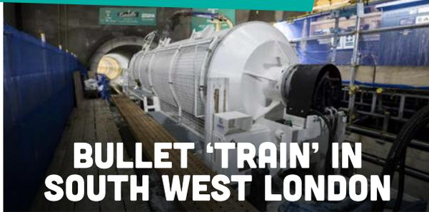
A bullet 'train' is hard at work on the secondary lining in the connection tunnel between Dormay Street and Carnwath Road, where it meets the main super sewer tunnel. The bullet which was manufactured in Germany weighs 11 tonnes when empty and 30 tonnes when full of concrete. It is being used to carry the concrete that will form the secondary lining of the connection tunnel.
