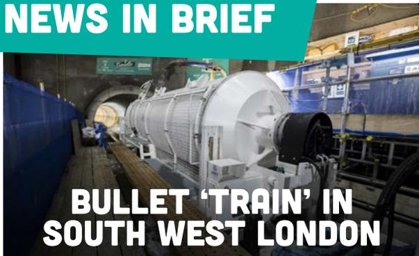
A bullet 'train' is hard at work on the secondary lining in the connection tunnel between Dormay Street and Carnwath Road, where it meets the main super sewer tunnel. The bullet which was manufactured in Germany weighs 11 tonnes when empty and 30 tonnes when full of concrete. It is being used to carry the concrete that will form the secondary lining of the connection tunnel.
