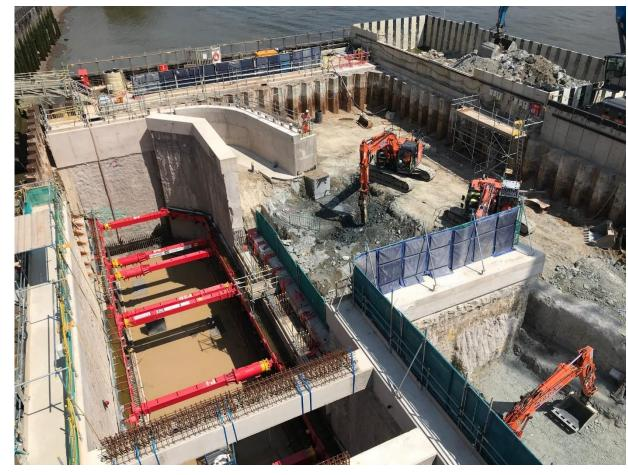
CSO base slab pour, installation of temporary props and excavation of the different hydraulic chambers
