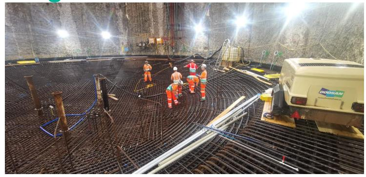
After the shaft excavation was completed, the base slab reinforcement was delivered by barge and installed in place
