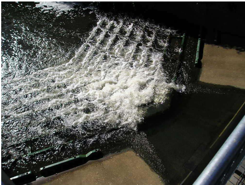
Figure 28 Isfield gauging station with structures designed to aid fish passage
