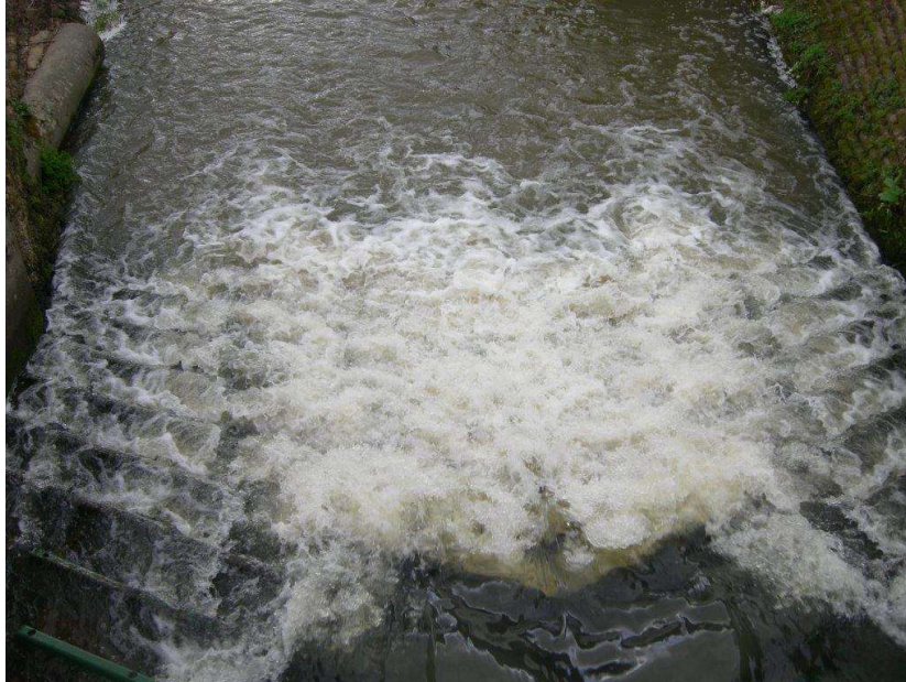
Figure 27 River Uck gauging station weir showing the use of square section block structures to aid fish passage. The spacing is approximately 40 cm and the section approximately 50mm
