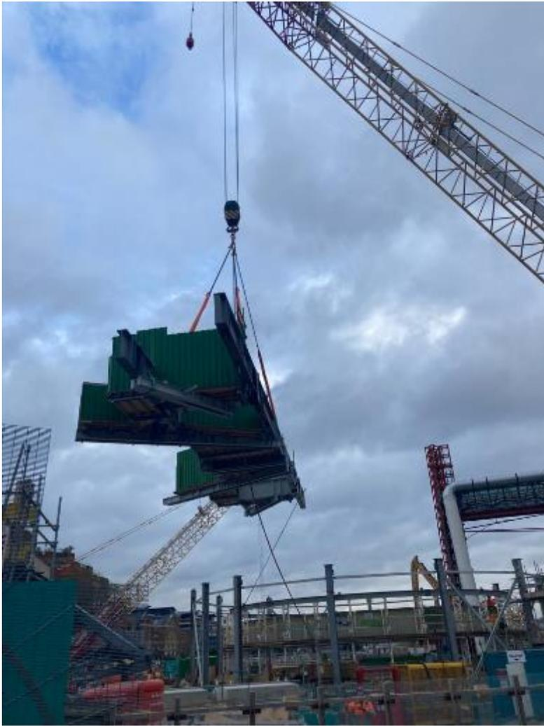
Slipform have commenced dismantling of the grillage and removal of box outs for shaft capping precast roof beams
