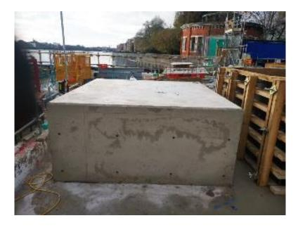
Commencing set up of the SCL batching plant – Silo base slabs
