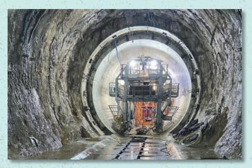
The secondary lining is needed to add extra strength to the tunnels, and will create a smooth surface over which the sewage can flow once the tunnel is operational in 2025.
