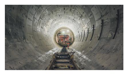
The full length of the super sewer is now linked following the breaking out of two giant grout plugs deep underground at Tideway's Blackfriars site.
