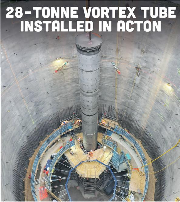
A 28-tonne vortex tube designed to carry sewage flows down and into the super sewer has been installed at Tideway's site at Acton Storm Tanks. The vortex (pictured above) will 'spin' the flows to protect the bottom of the shaft from erosion.
