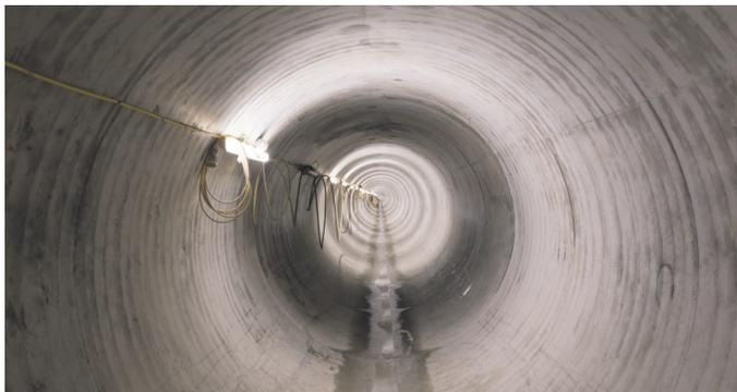
The 1.1km tunnel – known as the Frogmore Connection Tunnel – was excavated in two separate drives between 2019 and 2020, by a three-metre-wide tunnel boring machine (TBM) called Charlotte.
