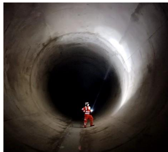
The main tunnel beneath the Thames
