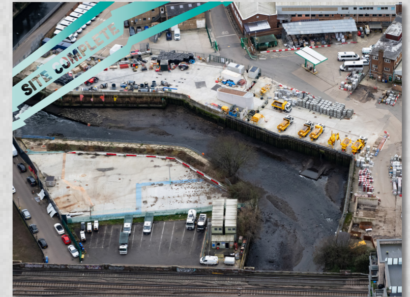
Aerial view of our Dormay Street site
