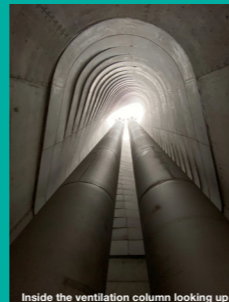
Inside the ventilation column looking up
