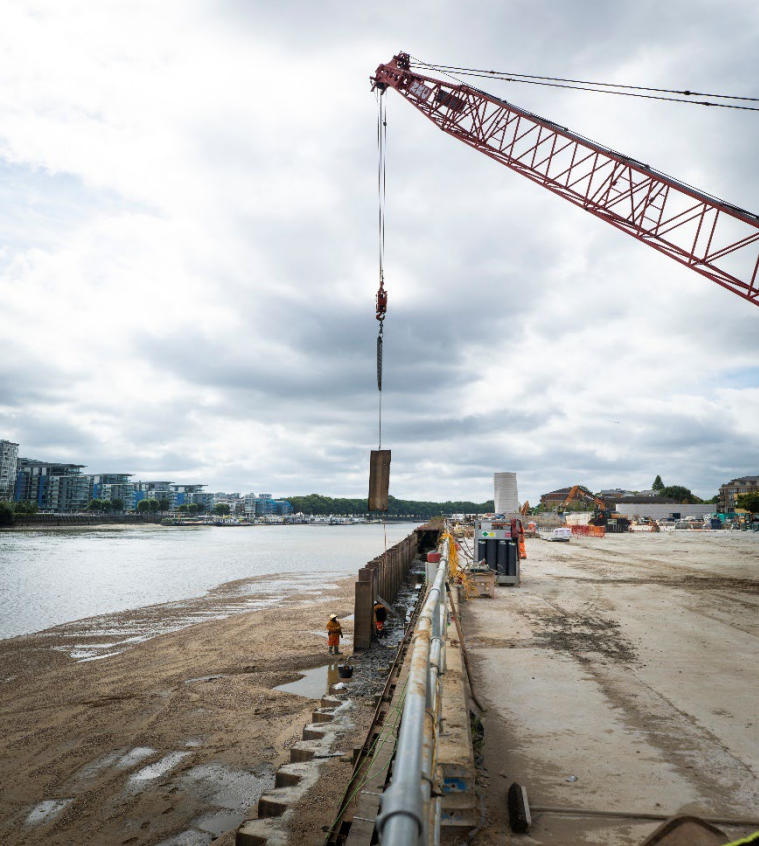
River wall works, removing piles and installing timber ecological enhancements. Due for full completion by: Oct 2024
