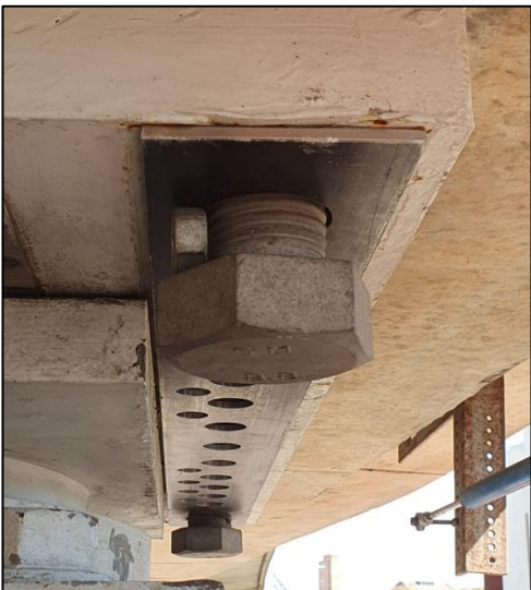
Pier P2 – with guide template
