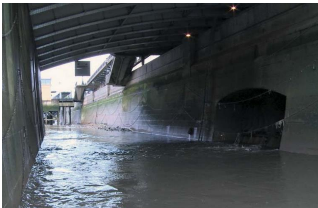
Figure 2-2 Fleet Main CSO outfall under Blackfriars Bridge
